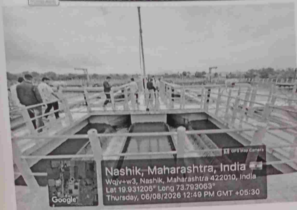
Explanation of Effluent Channels by Plant Manager
