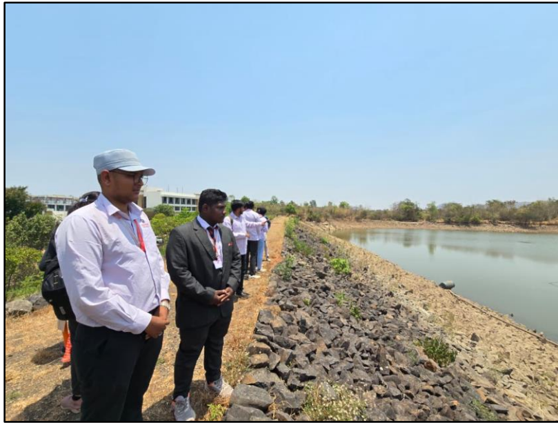
Figure 3: Civil Engineering students observing stone pitching technique implemented in the site for safe guarding the earthen slope
