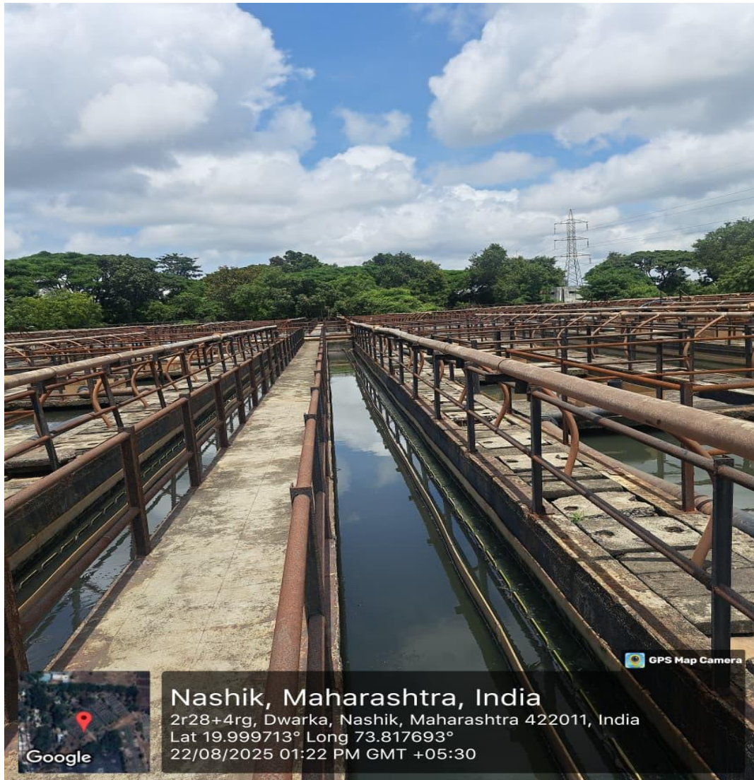
UASB Reactors
