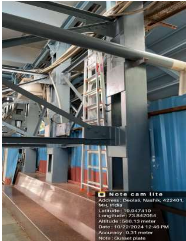
Channel section and gusset plates
